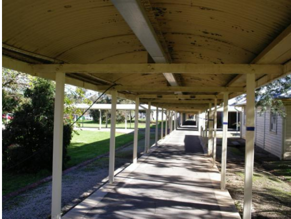
Picture 1: View of starting point for travel route
